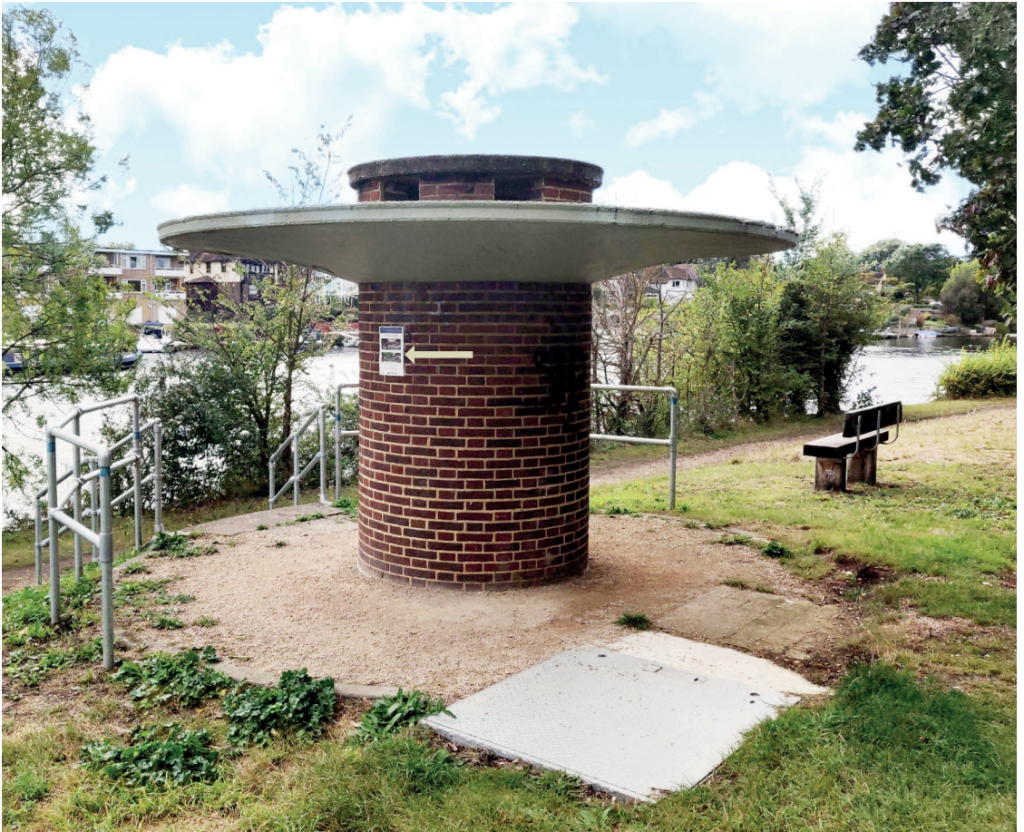
Above: The ventilator for the tunnel carrying the 2-foot gas main 16 feet below the bed of the river to Ditton. Covered by the hinged metal trap door, the access chamber is 14 feet in diameter and descends 40 feet to tunnel level. The arrow indicates the height reached by the river in the 1894 floods. Below: The original drawings as submitted.
