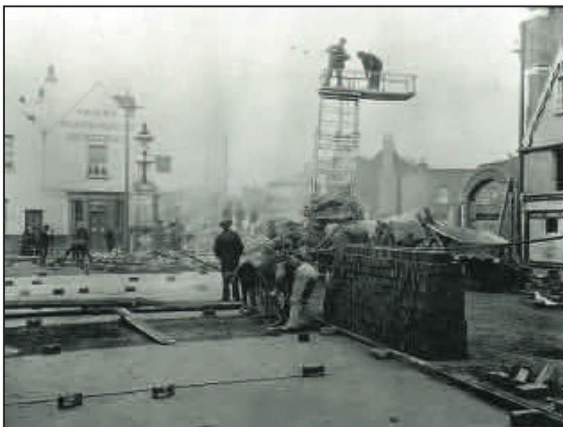
above: Even before demolition is completed, poles for the overhead wires are being erected and wood blocks for the road stacked ready to be laid.
